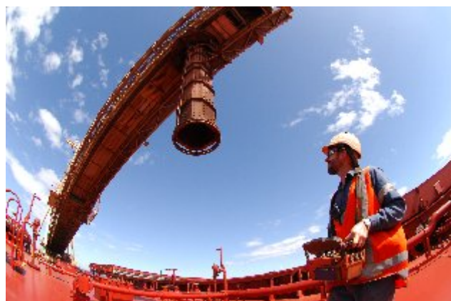
Figure 2: The adjustable chute on the shiploader means that the loading of iron ore can occur almost within the vessel's hold.
