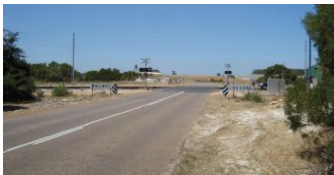
Above: Existing Sims Street road/rail crossing.
