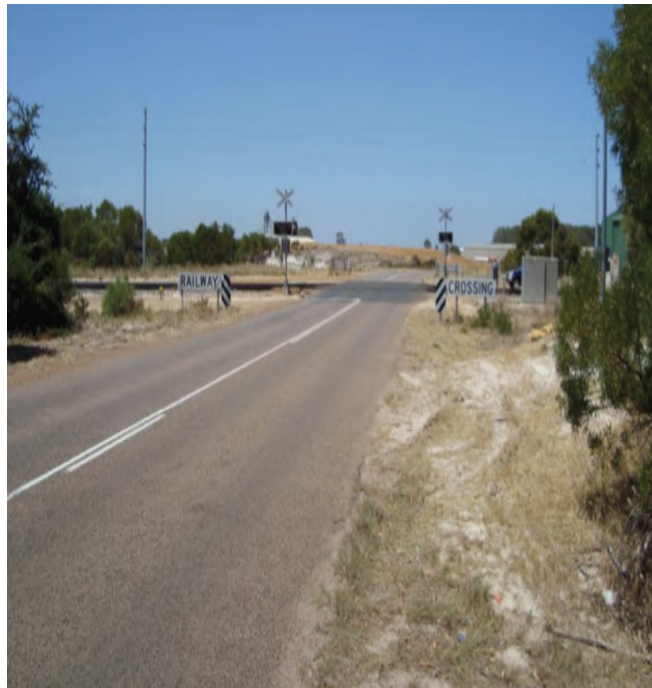
Above: Existing Sims Street road/rail crossing.
