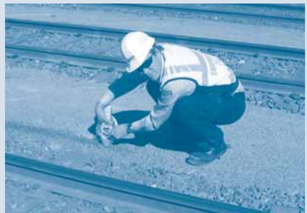
DEC officer using a hand held meter during preliminary testing for contamination along the rail line.
